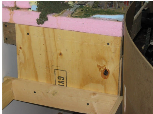
Photo 2 – A large trestle forced this drop in the benchwork height between this section and the one adjoining it. The pieces are held together by this plywood plate.
