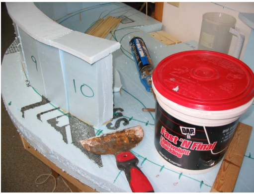
Photo 23 – Small gaps can be filled with lightweight spackling compound and a putty knife.
