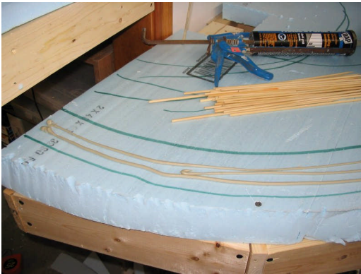
Photo 19 – Put down two heavy beads of adhesive.
