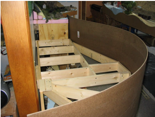
Photo 1 – Grid benchwork forms the foundation for the layout.
