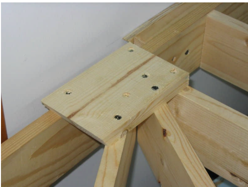
Photo 3 – A 1x4 gusset is used to attach radial joists at the curved end of the benchwork. This avoids the need for complicated geometry at the center of the radius.
